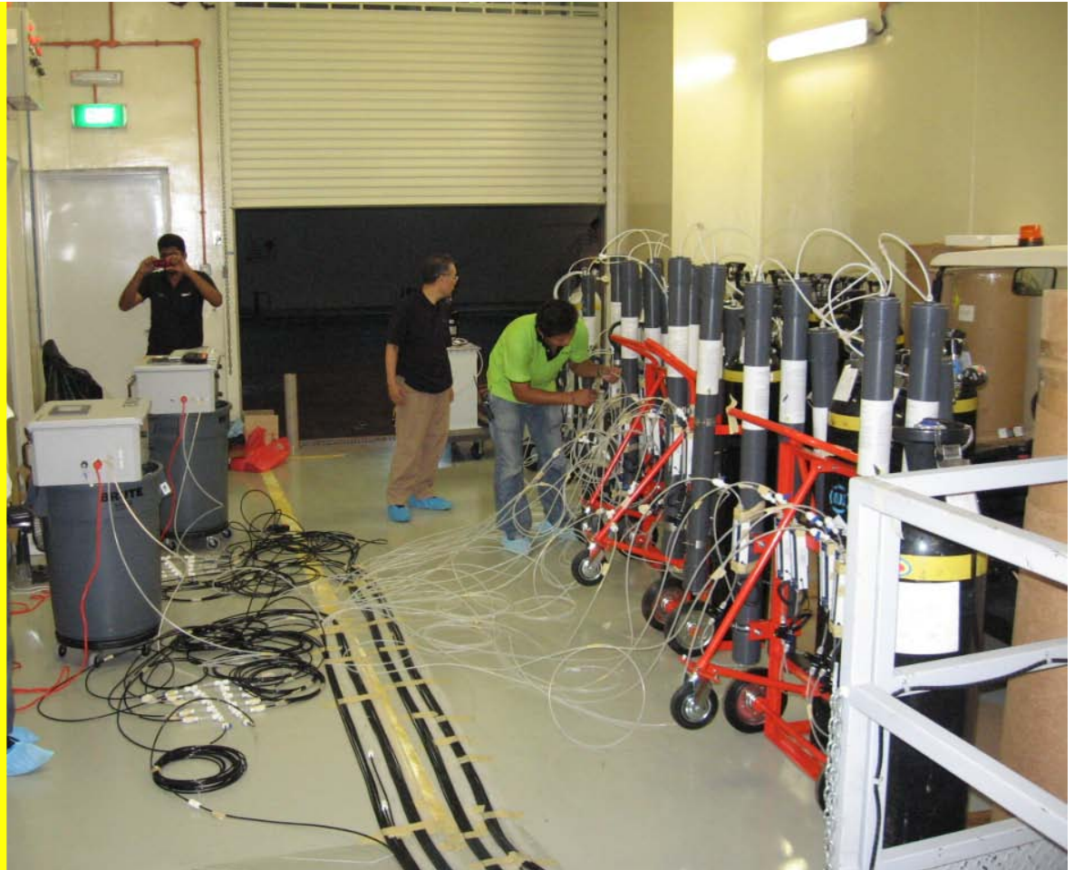
Disconnect and Remove Generators
